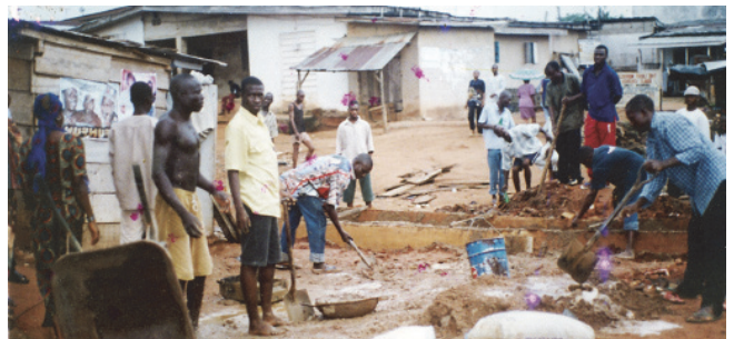
Community youth constructing a culvert after training on self help development
